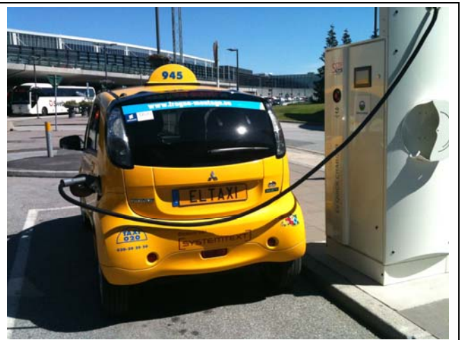
Figure 6. 50 kW DC fast charger (SGTE) at Arlanda Airport. Installation and Photo by Park & Charge i Sverige AB.
