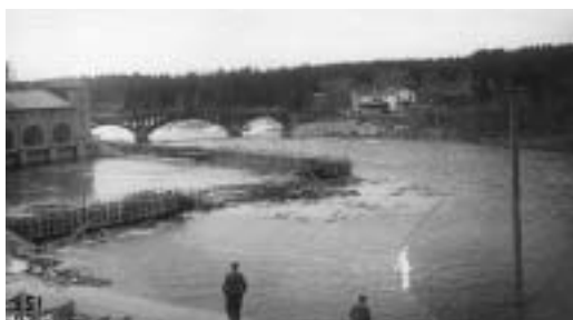
Älvkarleby hydro power station with the Karl XIII bridge. Construction began in 1910.
