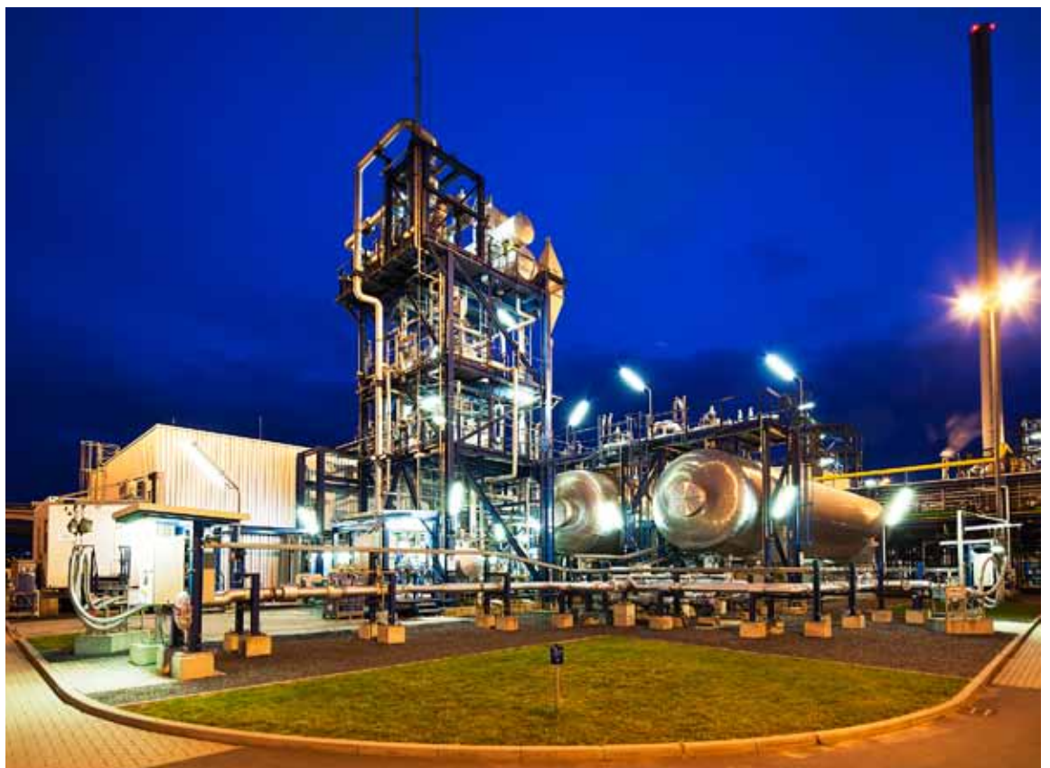
The CO 2 compression plant and intermediate storage tanks at the Oxyfuel pilot plant in Schwarze Pumpe.
