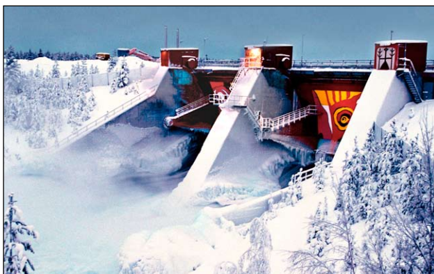
Akkats hydro power plant
