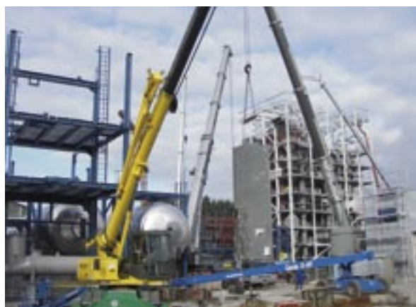
Assembly of the ASU coldbox
